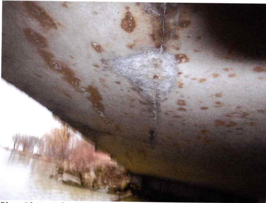
Photo #5 is at taken at the north end of the east beam that was damaged and cracked allowing water from the deck to cause additional deterioration. Notice how dry it is now (compare with the wet rusty condition seen on the bottom of the beam in the previous report).
