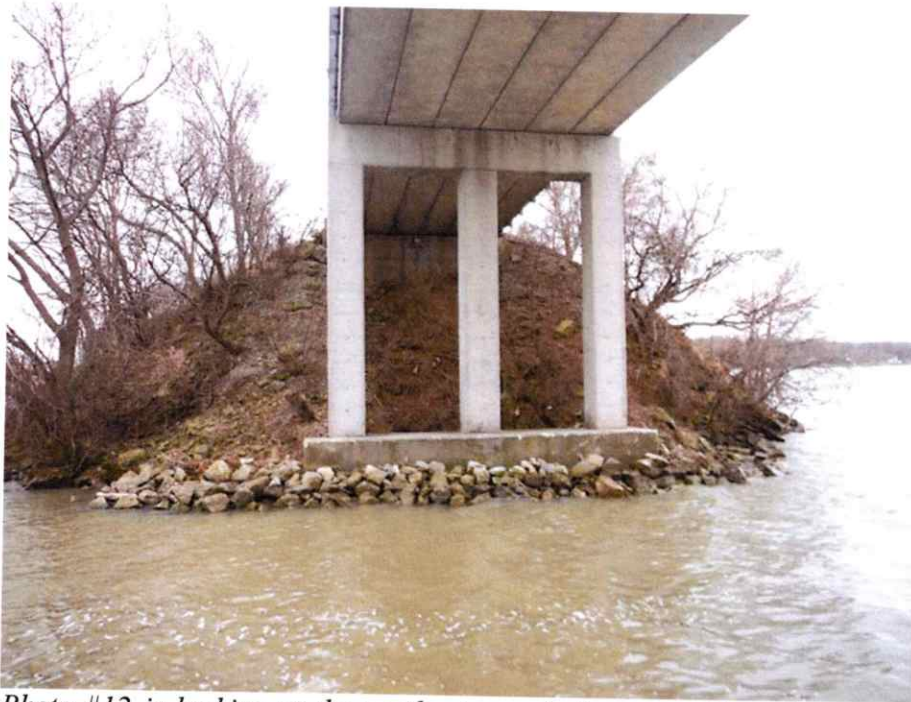
Photo #12 is looking at the south pier and abutment. Note the steepness of the embankment slope. The rock channel protection is in good condition. The vines and brush have been sprayed.
