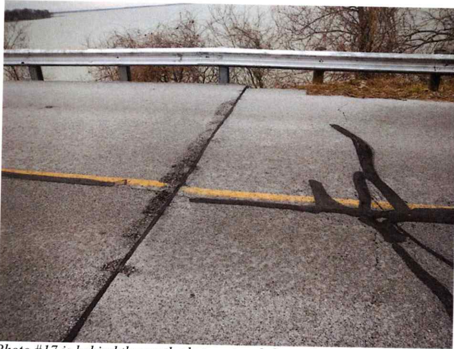
Photo #17 is behind the north abutment and shows the embankment settlement.
