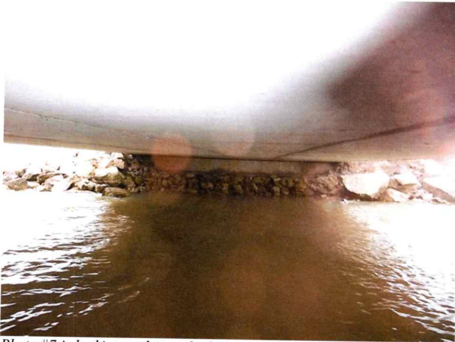
Photo #7 is looking at the north abutment. The dark spots seen on the abutment breast wall just appear to be staining from previous water leakage.
