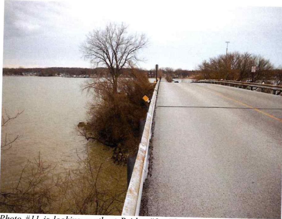
Photo #11 is looking north at Bridge #3. The asphalt is in good condition and there are no reflective cracks from the box beam joints seen in the pavement at this time.
