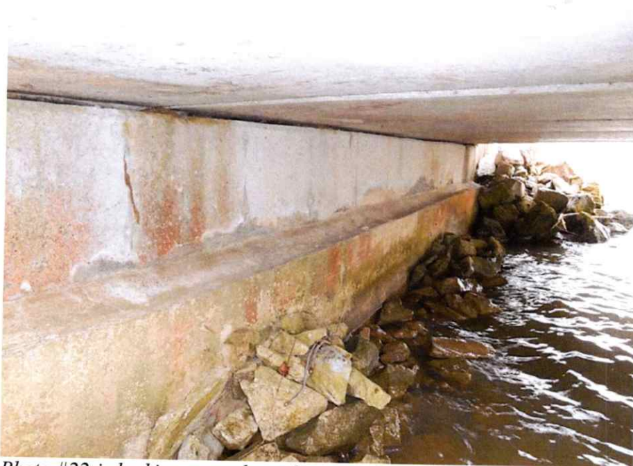
Photo #22 is looking west along the south abutment. The repair work is visible and it is still in good condition.
