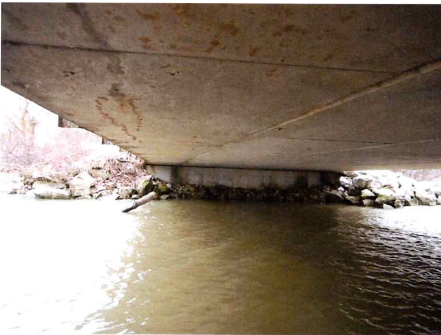
Photo #3 is looking at the south abutment. The dark spots seen on the abutment breast wall just appear to be staining from previous water leakage.
