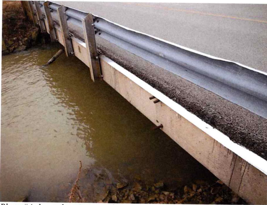
Photo #4 shows the missing railing post near the end of the east side that should be replaced.
