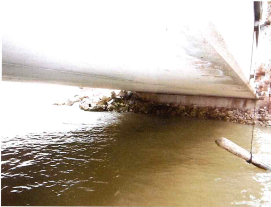
Photo #2 is looking north along the east side of the bridge. Note how dry the beams and abutments are. The waterproofing seems to be working well.
