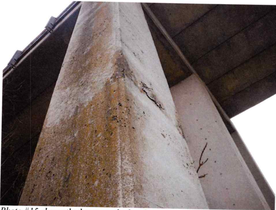
Photo #15 shows the honeycombed and spalling concrete at the north pier. There does not seem to be much change from previous inspections.
