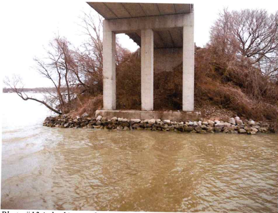
Photo #13 is looking at the north pier and abutment. The steep embankment is very uneven and eroded. The rock channel protection is also in good condition here. The bottoms of the beams in all spans appear to be dry.
