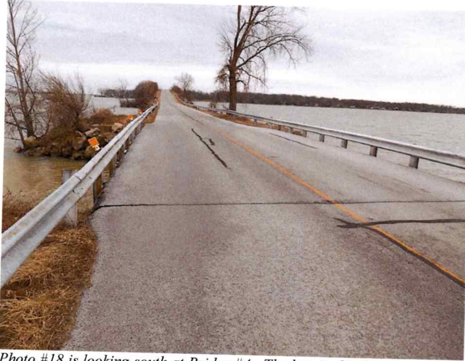
Photo #18 is looking south at Bridge #4. The longitudinal sealer seen on the deck is apparently over one of the beam joints.
