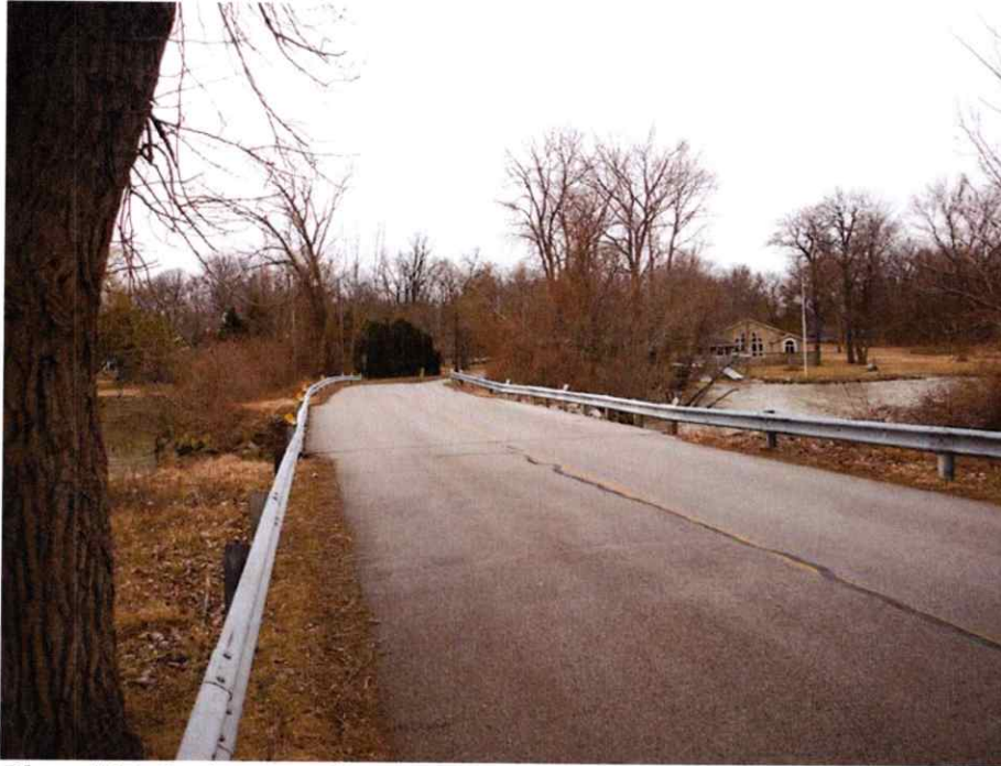
Photo #1 is looking south at Bridge #1. The asphalt is in good condition and there are no reflective cracks from the box beam joints seen in the pavement at this time.
