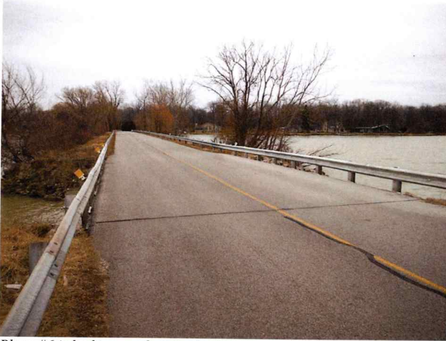
Photo #6 is looking south at Bridge #2. The asphalt is in good condition and there are no reflective cracks from the box beam joints seen in the pavement at this time.
