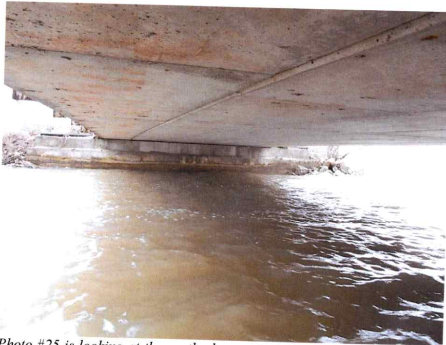
Photo #25 is looking at the south abutment. Little rock channel protection is still visible above the water. Note that the bottom of the beams and the face of the abutment are dry now with the new waterproofing.
