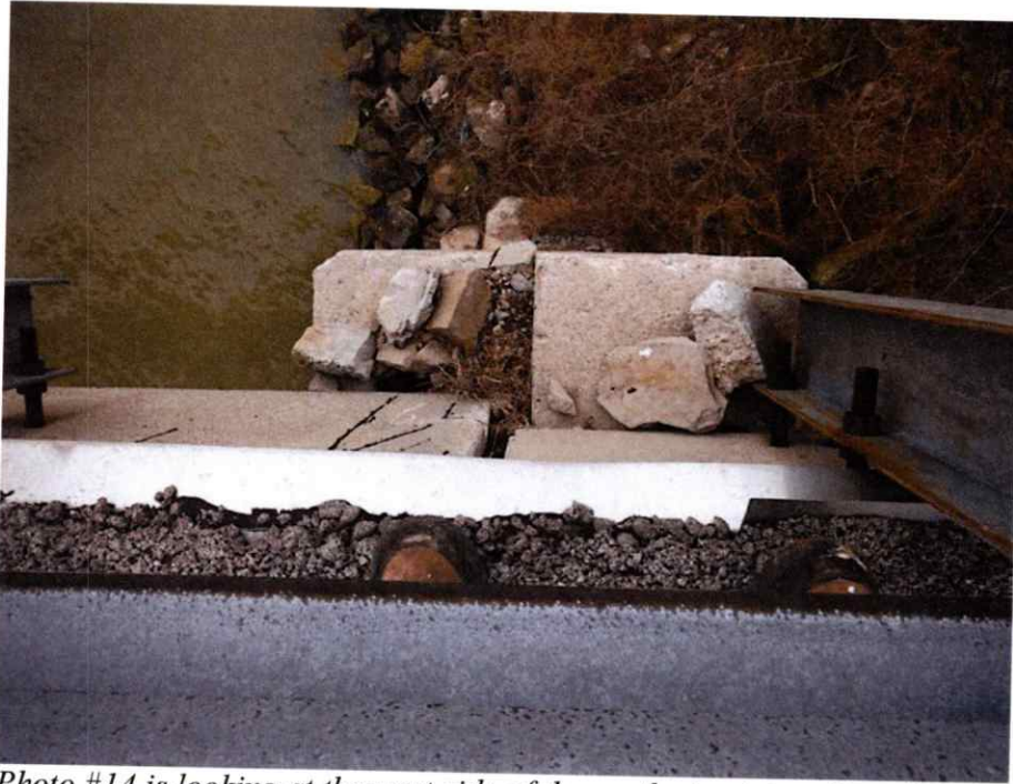
Photo #14 is looking at the west side of the north pier joint. Note that there is no concrete in the joint here between the beams. The other locations still have the concrete in the joint or have been patched.
