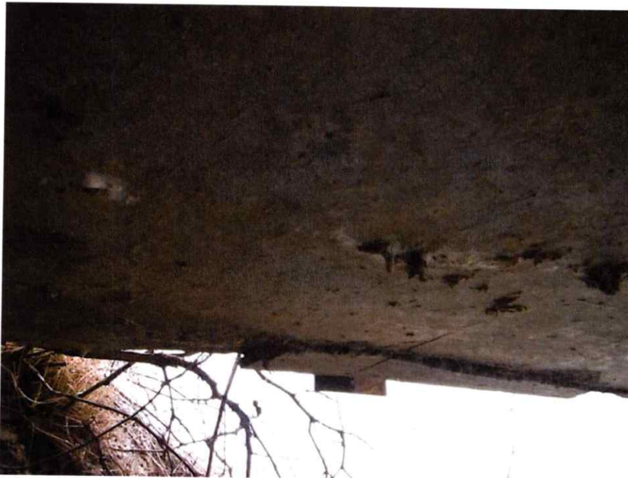
Photo #10 shows the same east beam damaged area looking at it from under the bridge. The beam bottom is now dry after the installation of the waterproofing.
