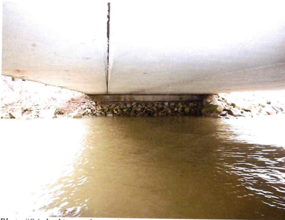
Photo #8 is looking at the south abutment. Note how dry the beams and abutments are. The waterproofing seems to be working well.
