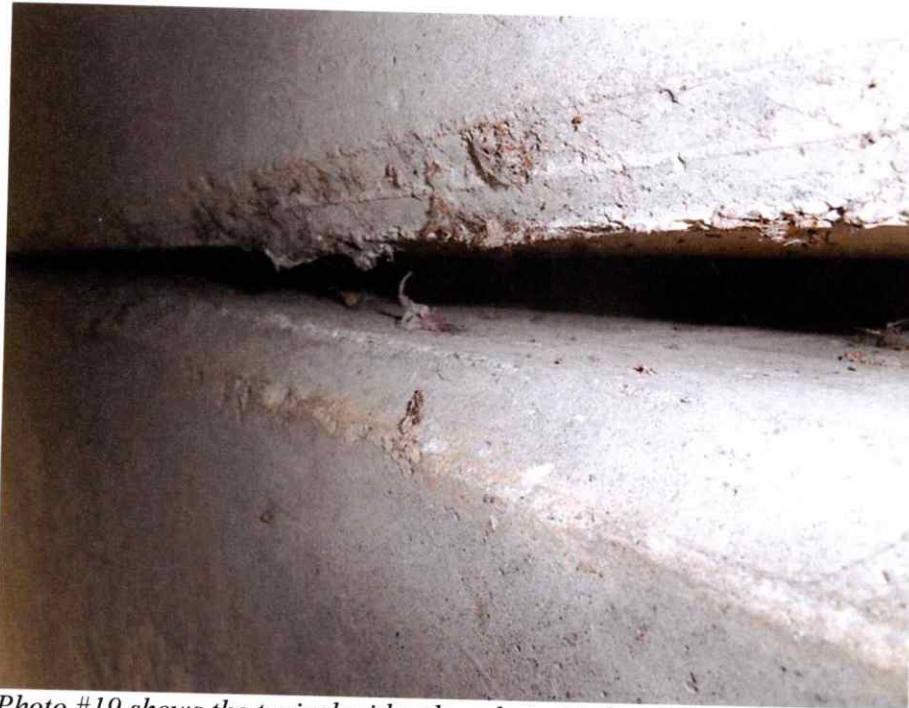
Photo #19 shows the typical wider than desirable box beam joints,
