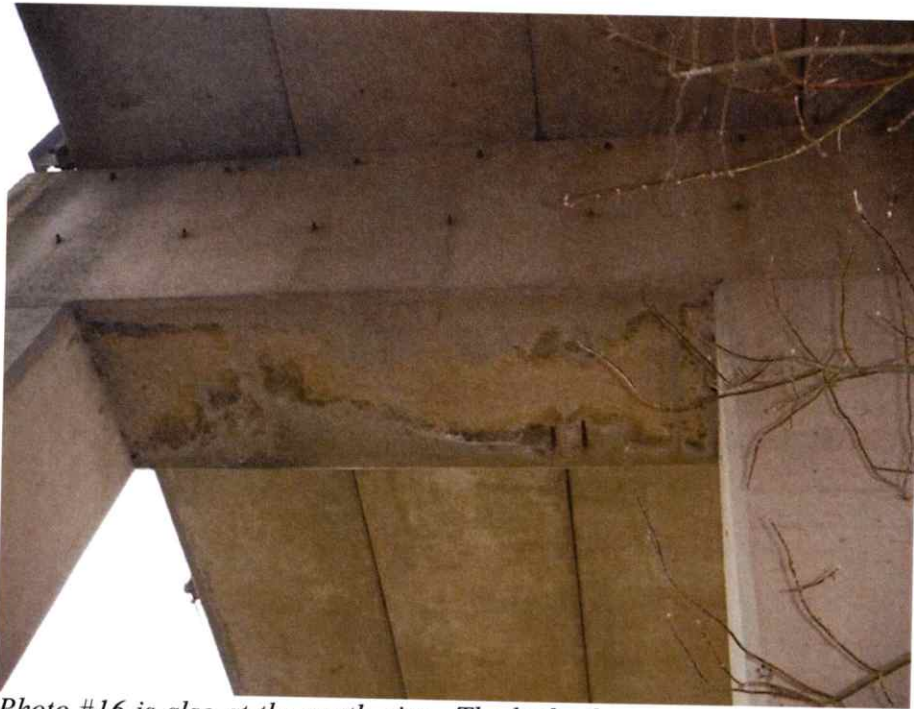
Photo #16 is also at the north pier. The lack of concrete cover on the bottom of the pier cap is the cause of the exposed bars here.
