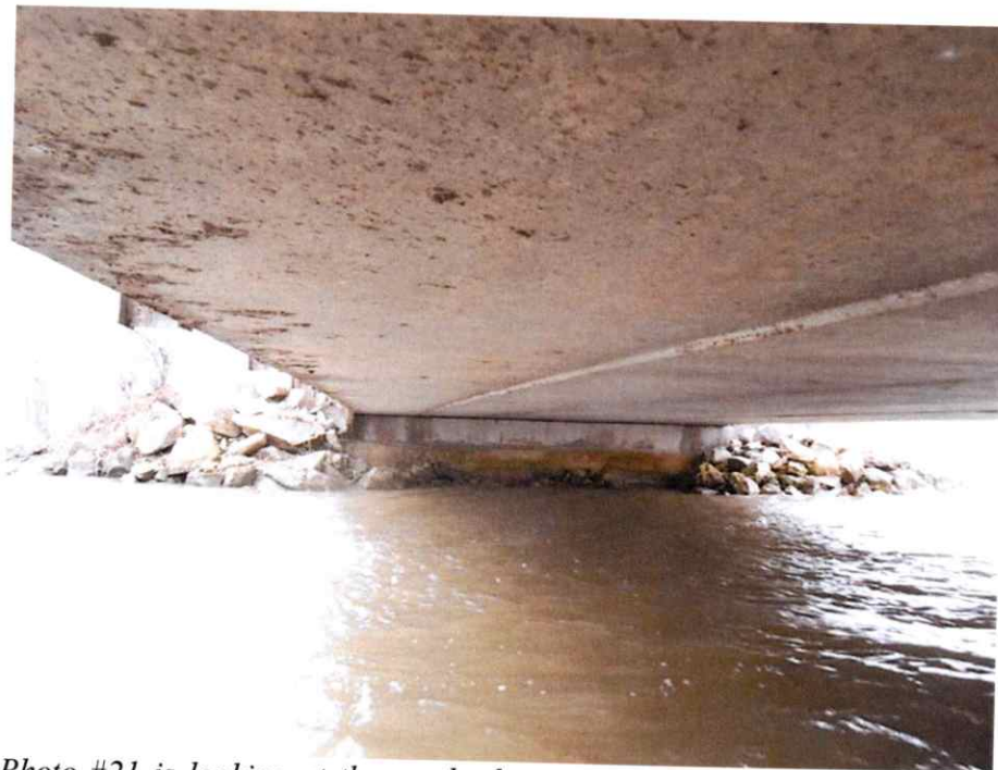
Photo #21 is looking at the south abutment. Some of the rock channel protection appears to have slumped down in front of the abutment breast wall.
