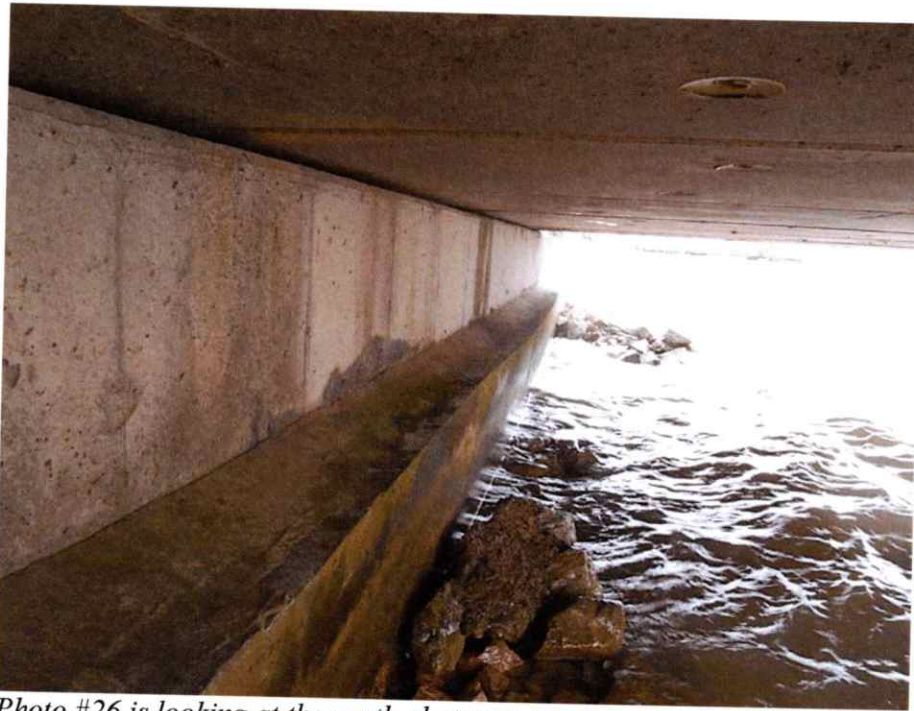
Photo #26 is looking at the north abutment concrete repairs which appear in good condition.
