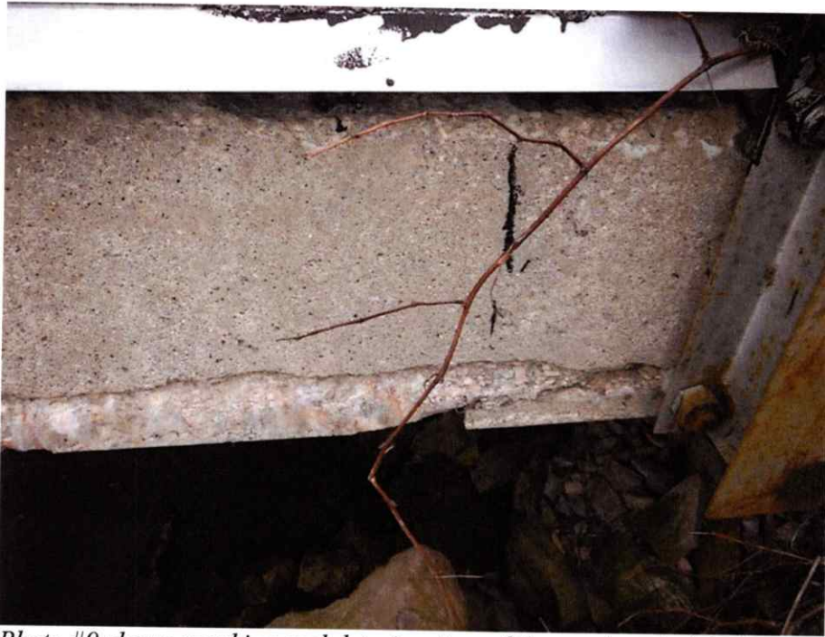
Photo #9 shows cracking and deterioration of the north end of the bottom of the east beam. This damage apparently resulted from an impact to the railing.
