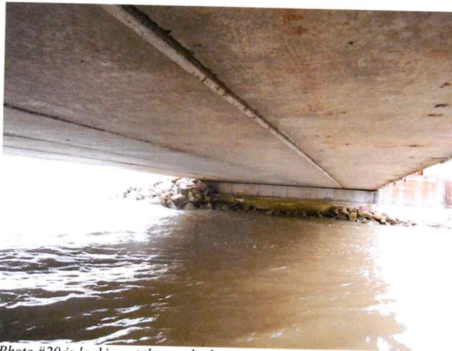
Photo #20 is looking at the north abutment. Adding additional rock channel protection would be desirable.
