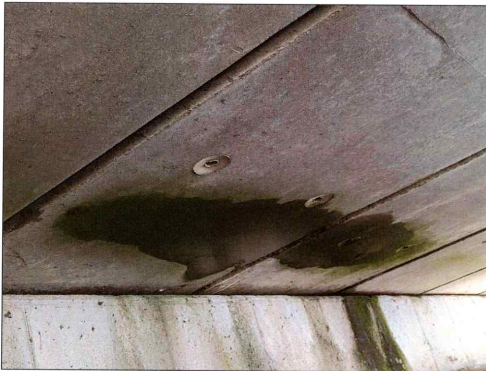
Picture 26: Leaking beam joint at north abutment (Bridge 5). (This leak was not present during the previous inspection)
