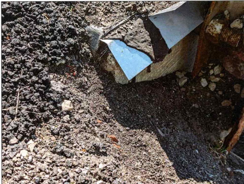
Picture 24: Erosion at northwest corner (Bridge 5).
