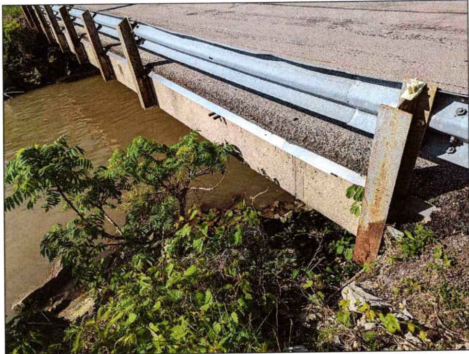
Picture 4: Missing railing post at northeast (Bridge 1).
