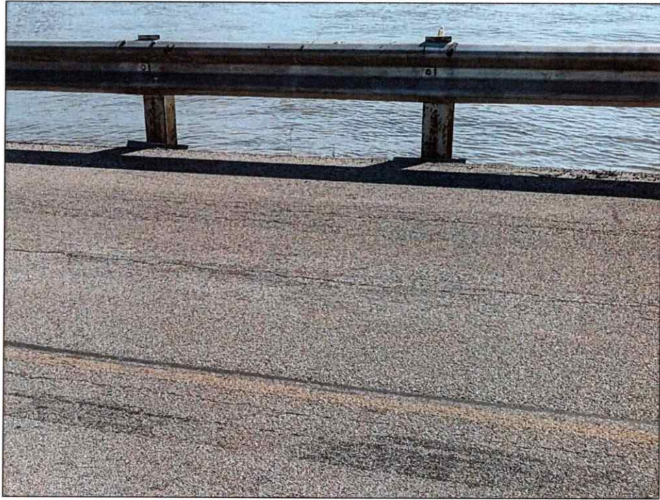
Picture 8: Cracks in the wearing surface (Bridge 2).
