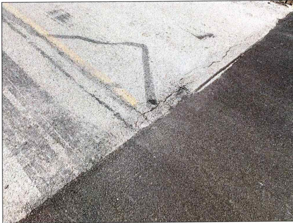
Picture 29: Transverse cracks at north transition (Bridge 5).
