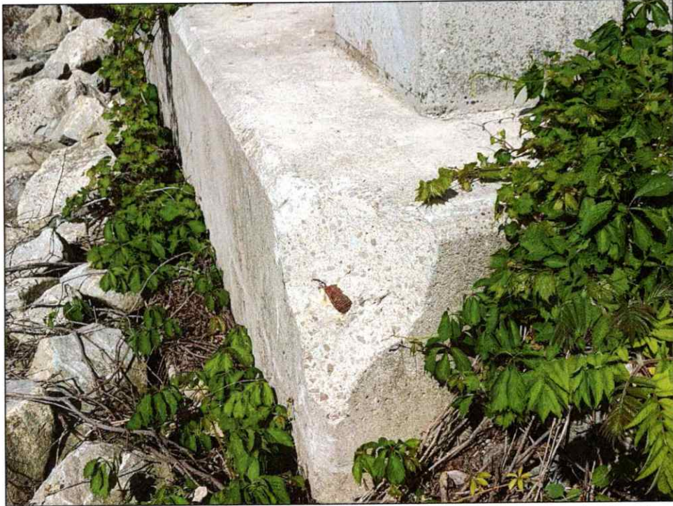
Picture 15: Spall with exposed rebar at southeast corner of the north pier (Bridge 3).
