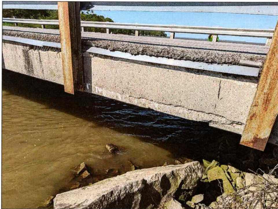
Picture 9: Damage on edge of east beam at north end (Bridge 2).
