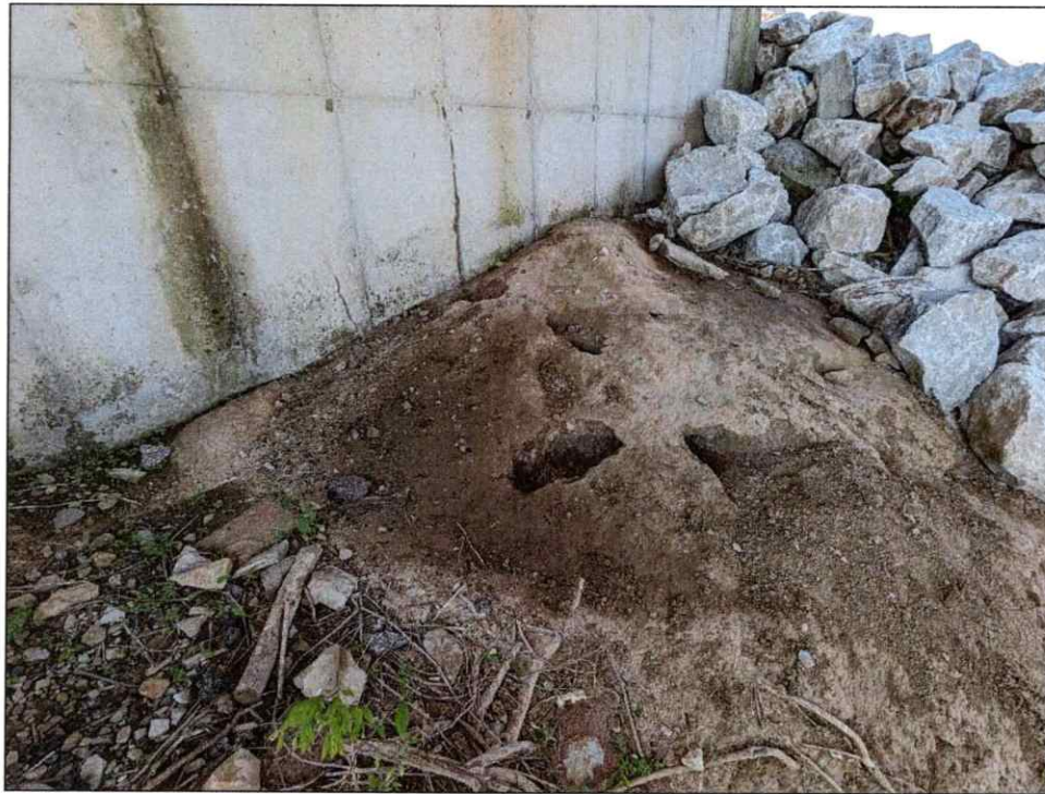
Picture 17: Animal holes at top of south slope (Bridge 3).
